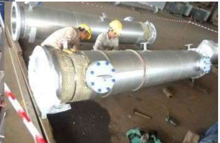
Insulation in progress for Glycol still columns.
